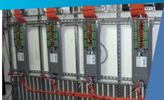
The Installation Frames installed in a dimmer room with all wiring completed and tested.
