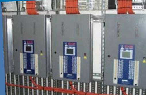
Hanging and commissioning 96 channels of dimmers onto the Installation Frames took less than 30 minutes.
