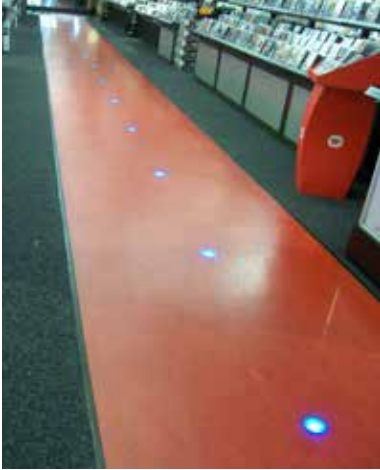
Probably Sydney's oldest LED Lighting installation of it's type, and Digilin's first
