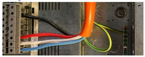
5. Terminate the supply group of the wiring loom into the left-hand side of the terminals. Refer to 2.4.4 Wiring loom for more information.
