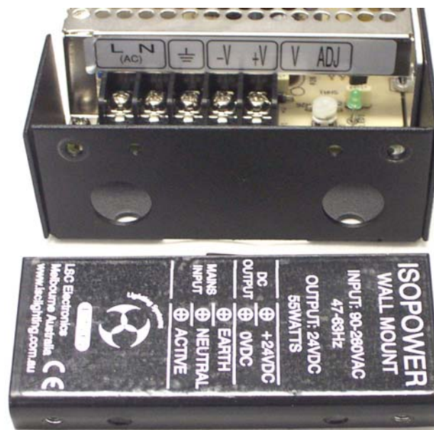
ISPW connections with cover removed
